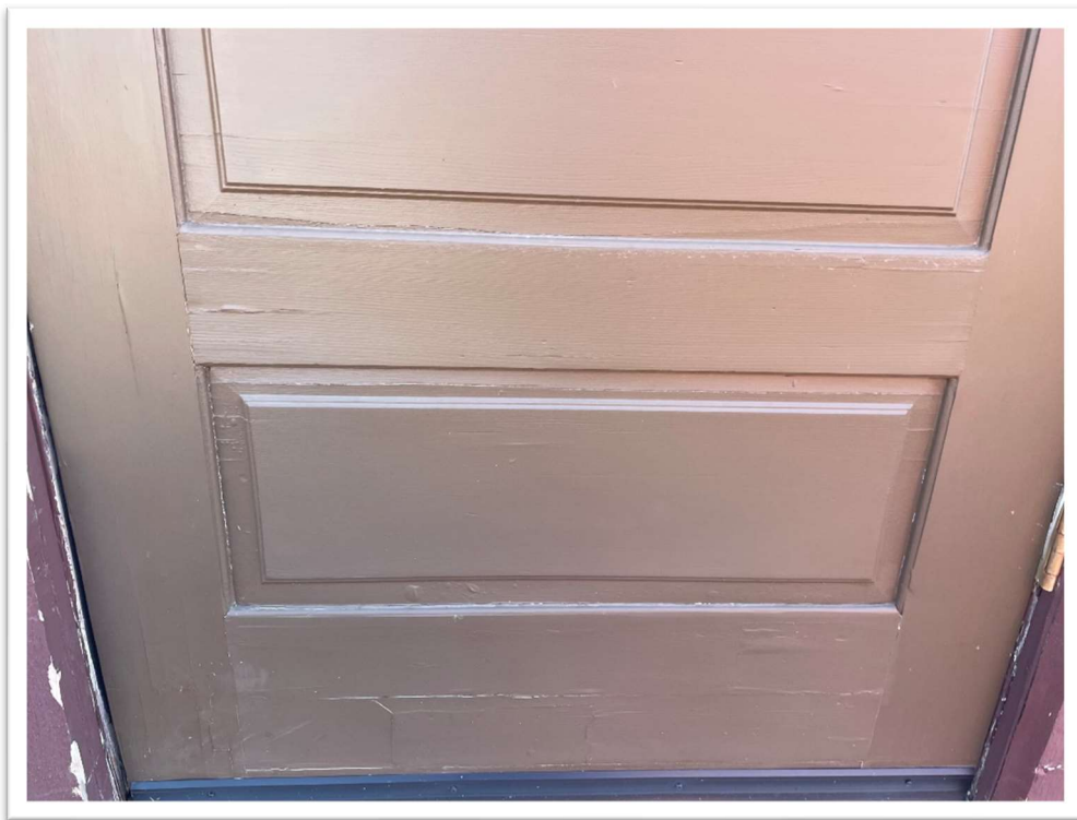
West door and 2023 water damage, June 22, 2023
