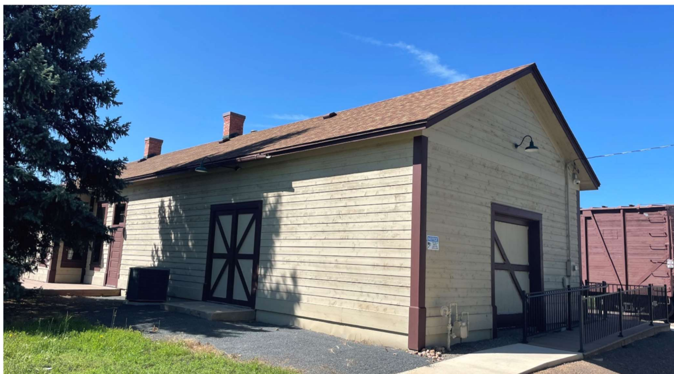
Northeast Corner, June 22, 2023
