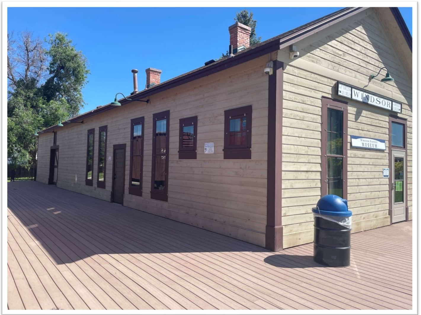
Southwest corner, proposing adding gutter to west side of building, June 22, 2023
