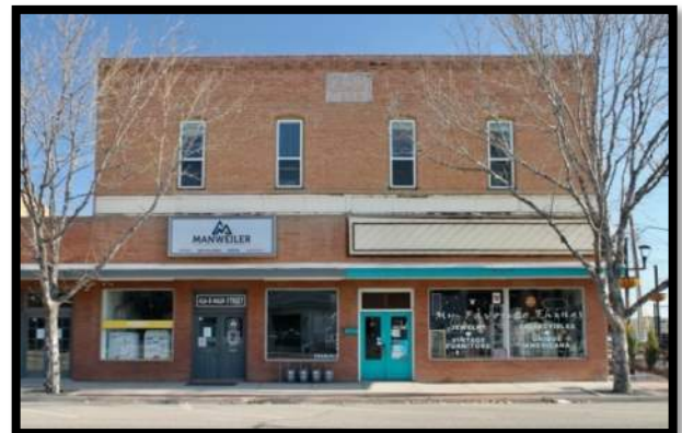
414 Main St., Windsor Mercantile and Odd Fellows Hall, Built 1898
