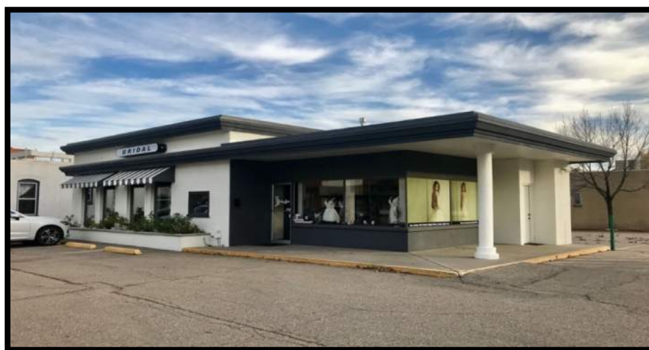
Frontier-Husky Gasoline Station, 529 Main St.
