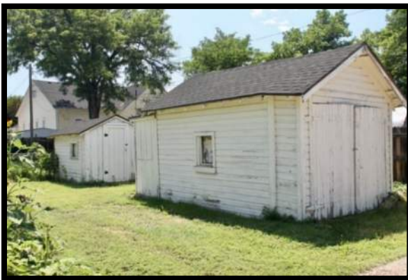
Single-Wide Garage and Shed Wood-Frame Construction
