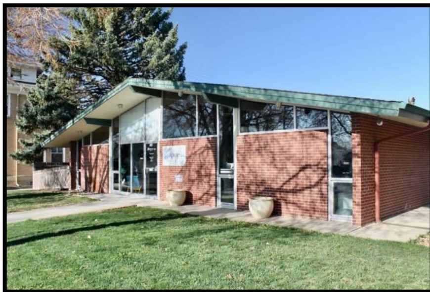
Windsor Library, 214 5 th St., Built 1960-1961
