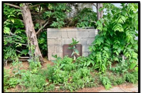
Likely Trash Incinerator Cinder Block Construction
