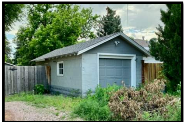
Single-Wide Garage Concrete Block on Stone Foundation
