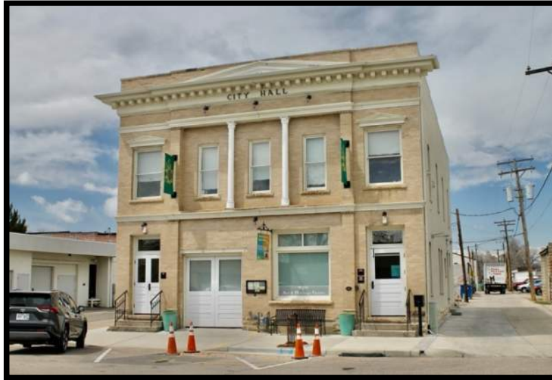
Historic Town Hall / Current Windsor Art & Heritage Center, 116 5th St.
