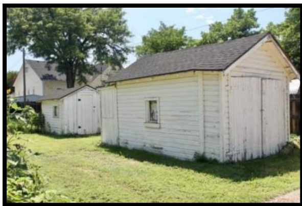
Single-Wide Garage and Shed Wood-Frame Construction
