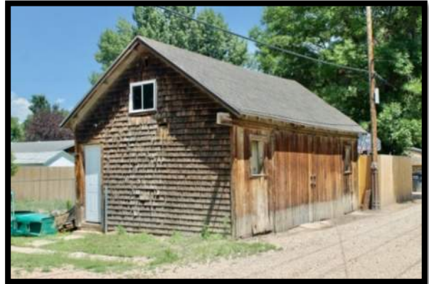
Oversized Single-Wide Garage Sliding Wood Doors on Side Entry
