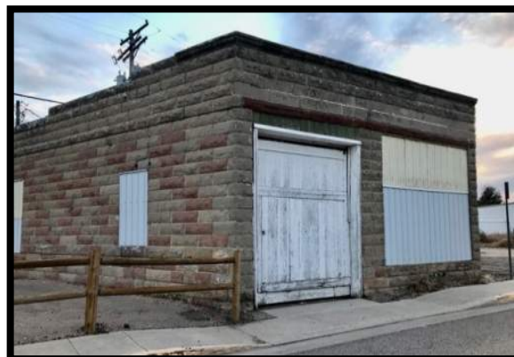
Lot 8, Block 6, Facing the Railroad Corridor
