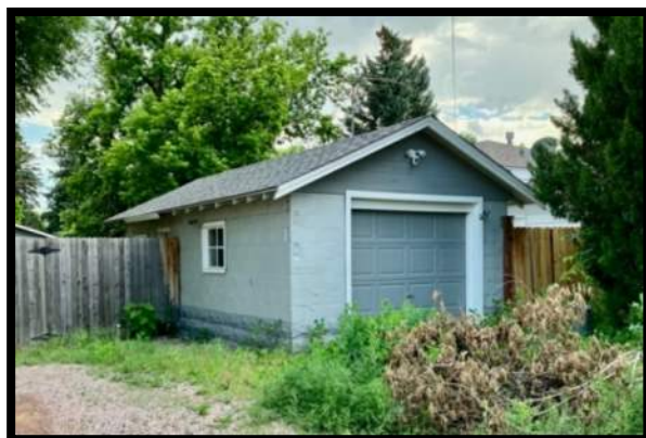
Single-Wide Garage Concrete Block on Stone Foundation
