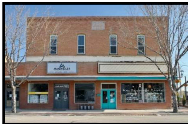
414 Main St., Windsor Mercantile and Odd Fellows Hall, Built 1898
