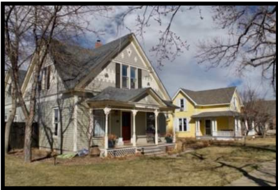
Houses in 400 Block of Walnut St.
