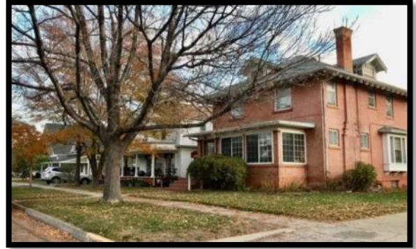
Houses in 400 Block of Walnut St.
