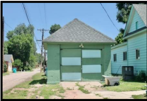
Single-Wide Garage Brick Walls and Hipped Roof
