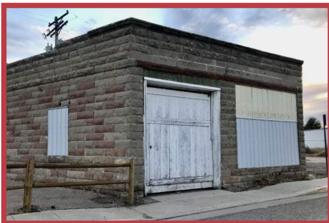
Lot 8, Block 6, Facing the Railroad Corridor
