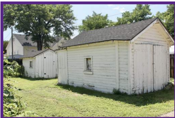
Single-Wide Garage and Shed Wood-Frame Construction
