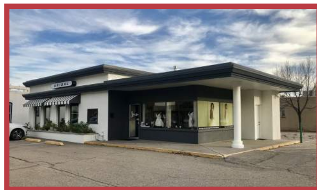
Frontier-Husky Gasoline Station, 529 Main St.
