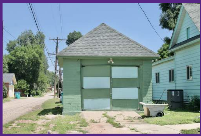
Single-Wide Garage Brick Walls and Hipped Roof
