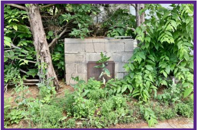
Likely Trash Incinerator Cinder Block Construction
