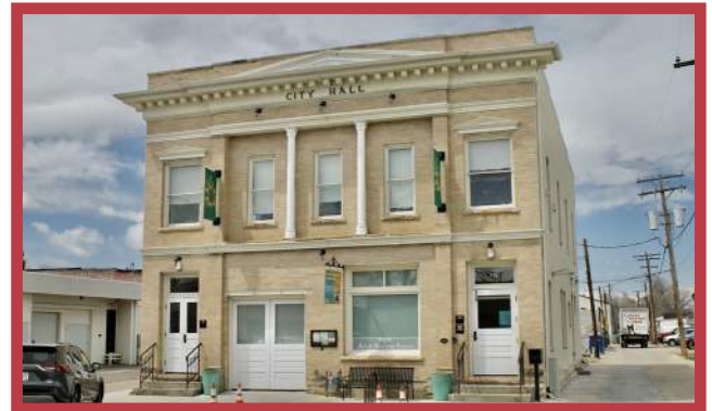
Historic Town Hall / Current Windsor Art & Heritage Center, 116 5th St.
