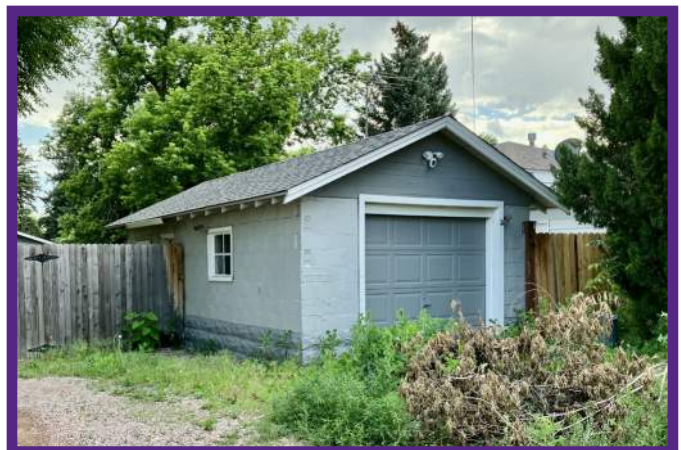
Single-Wide Garage Concrete Block on Stone Foundation
