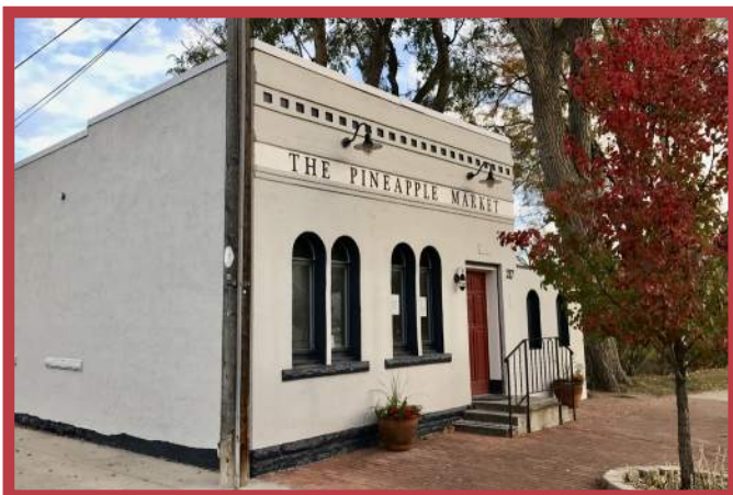
217 5th St., Mountain States Telephone & Telegraph Building
