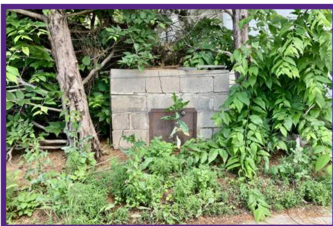
Likely Trash Incinerator Cinder Block Construction
