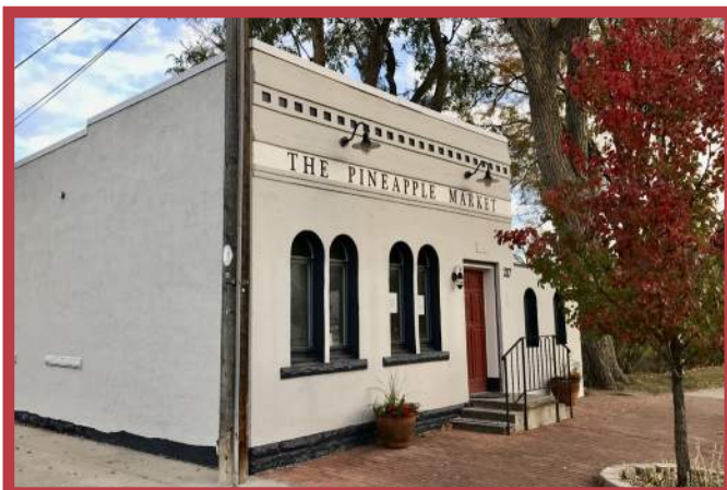
Mountain States Telephone & Telegraph Building, 217 5th St.
