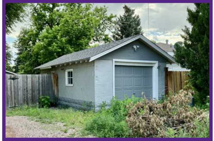
Single-Wide Garage Concrete Block on Stone Foundation
