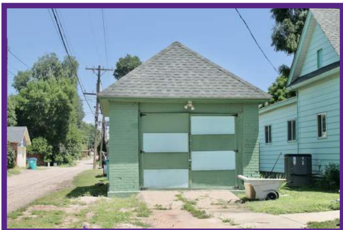
Single-Wide Garage Brick Walls and Hipped Roof
