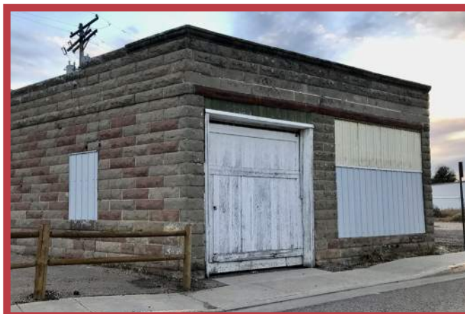
Lot 8, Block 6, Facing the Railroad Corridor
