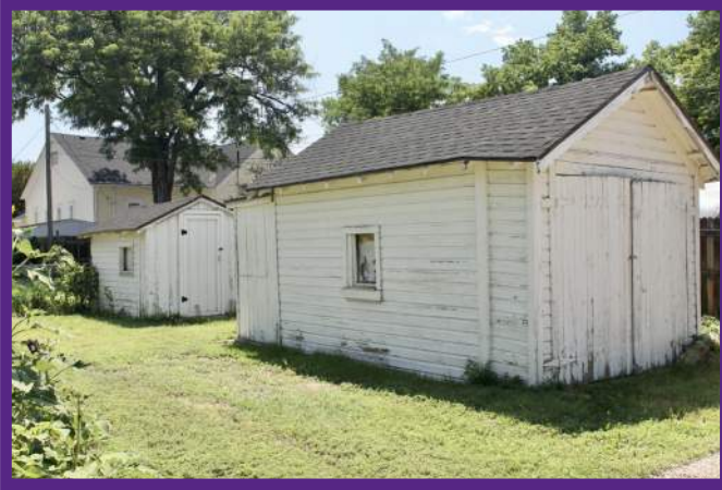
Single-Wide Garage and Shed Wood-Frame Construction
