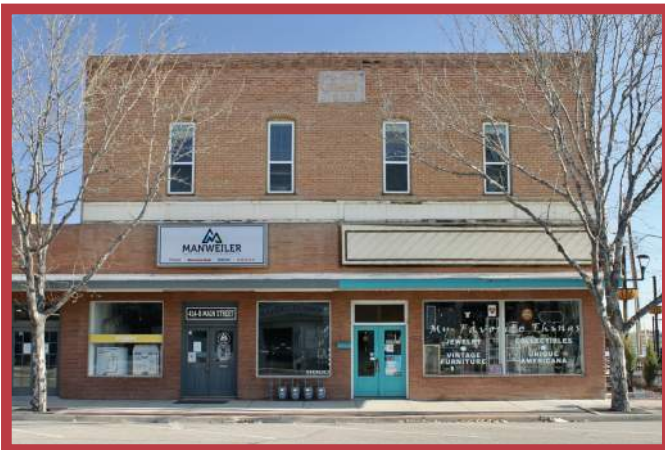
Windsor Mercantile and Odd Fellows Hall, 414 Main St.
