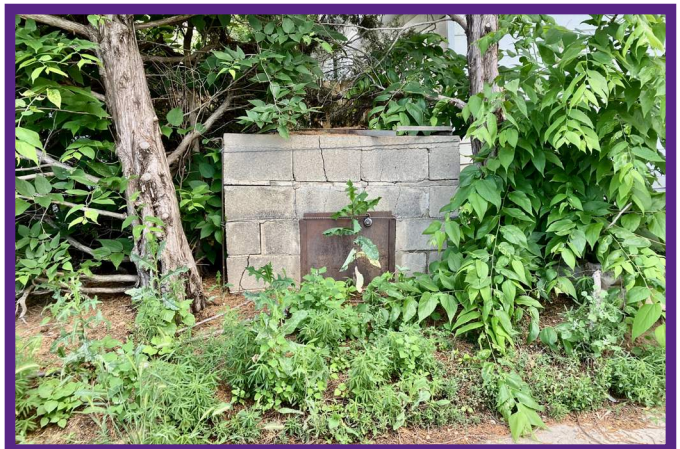
Likely Trash Incinerator Cinder Block Construction
