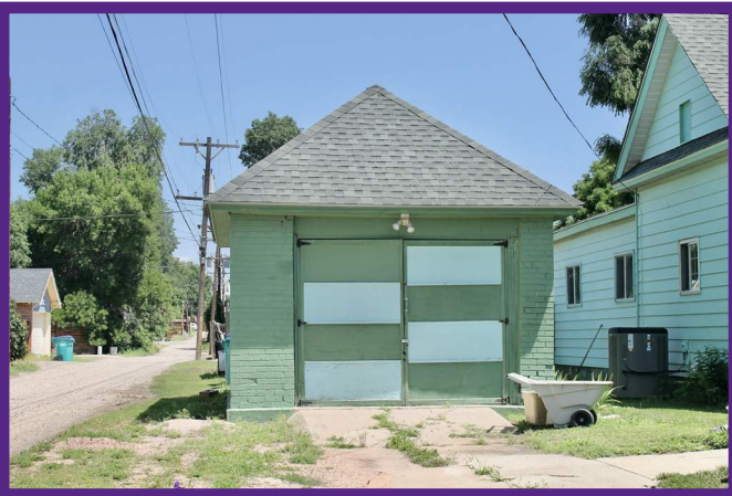
Single-Wide Garage Brick Walls and Hipped Roof
