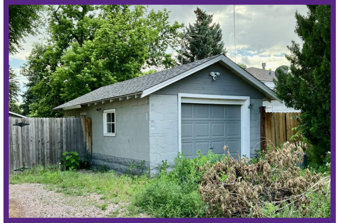
Single-Wide Garage Concrete Block on Stone Foundation
