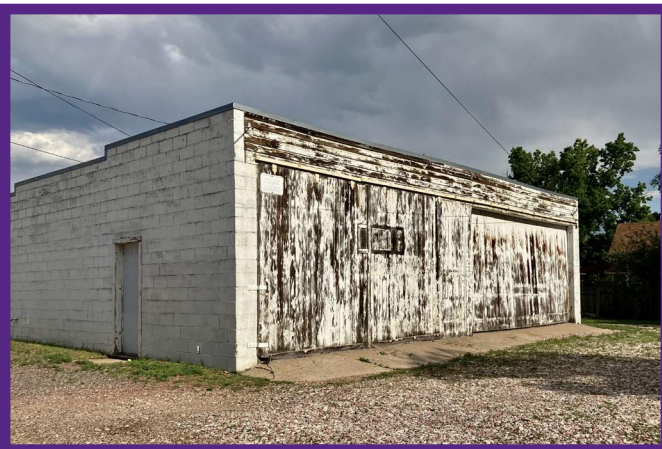
Large Shop Building Oversize Doors and Concrete Block Walls
