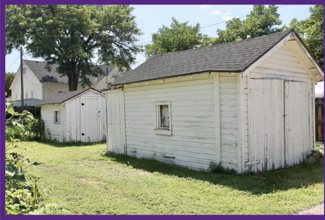
Single-Wide Garage and Shed Wood-Frame Construction
