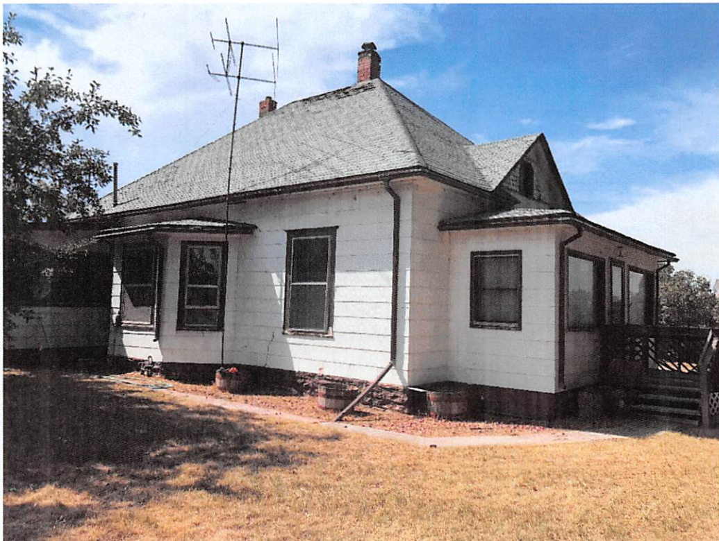
View from the southeast corner showing outline of roof and dormer.
