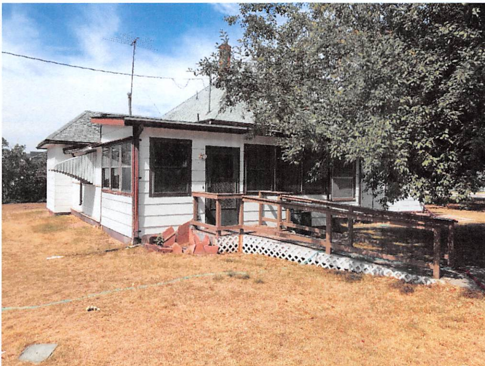
Enclosed porch addition on southwest corner of the house with shed roof. The ramp was added in the 90s while Norman Jacoby was still living in the house at the end of his life.
