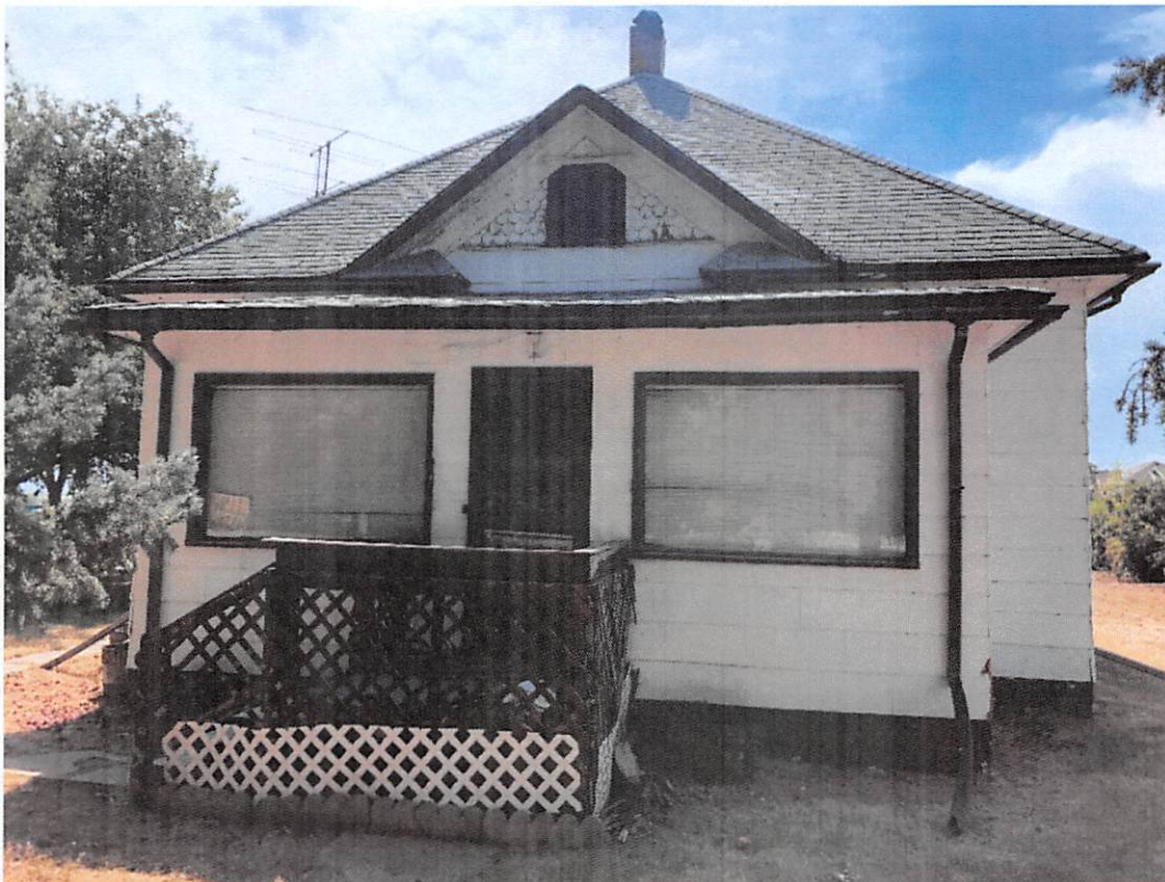
Front (east) of house with original porch that has been enclosed and stairs added. The dormer window of the second half-story is visible with original “gingerbread” work.
