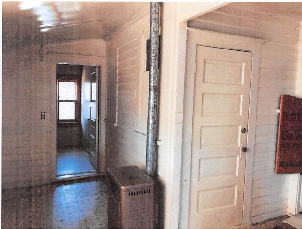
Interior of later additions showing the door leading to the cellar (right) and the door to the first addition.
