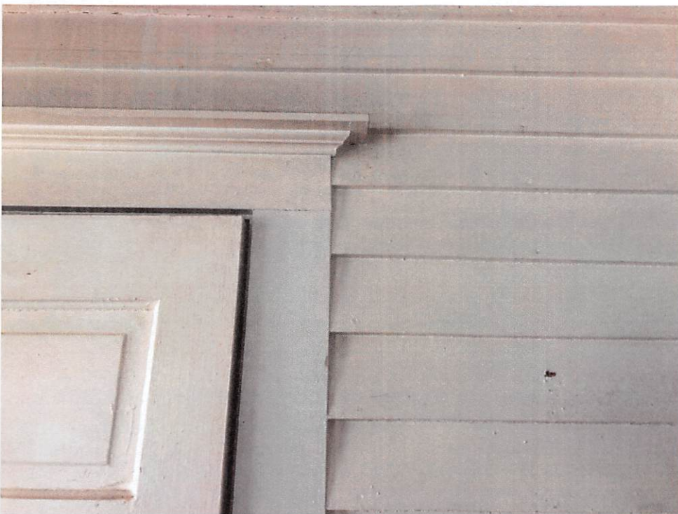
Original shiplap siding and door trim still visible inside the later additions. This was originally the exterior of the house.
