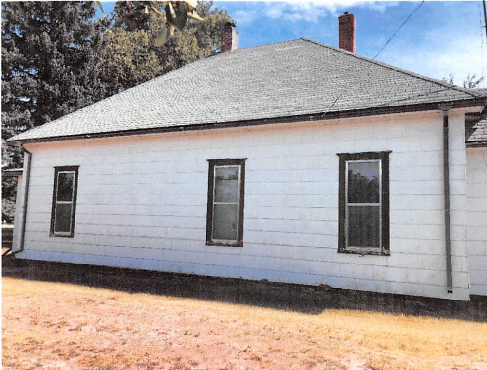
North side of the house with hip roof visible.
