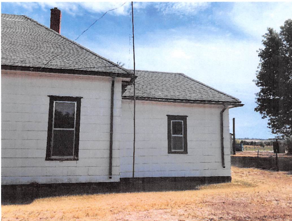
First addition built on to the north end of the west side of the house. The builder attempted to match the roof and window styles.
