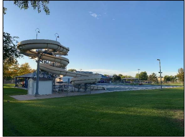
Pool facility slide
