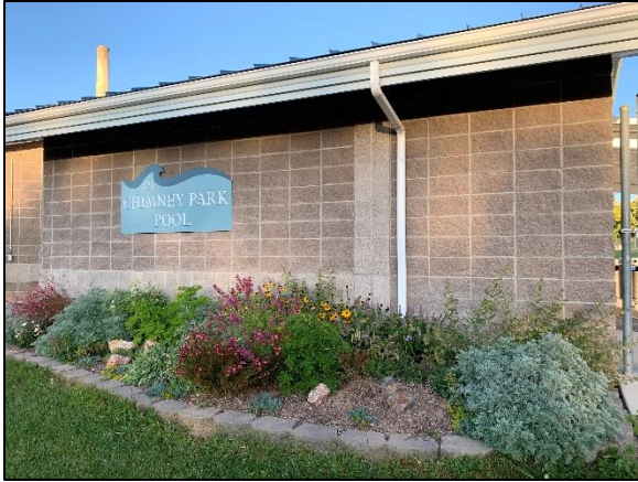
Chimney Park Pool Bathhouse
