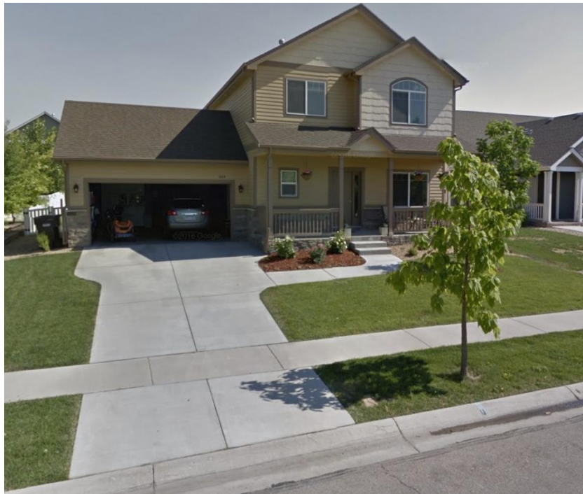
Limited Access: recessed garage. New Windsor
