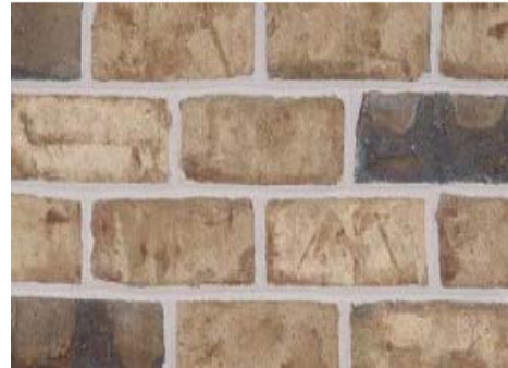
brick façade & wainscot
