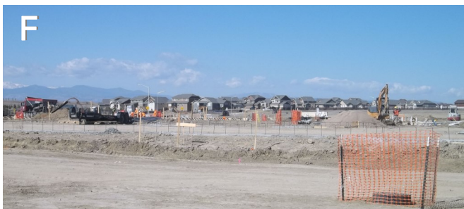
F South Hill 6th—The Falls Apartments—120 unit age restricted apartment complex under construction
