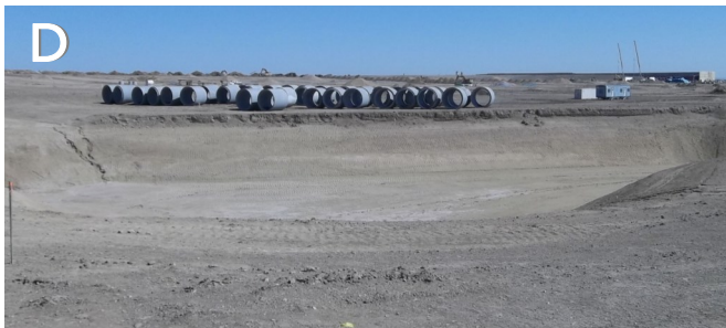
D Raindance Subdivision 1st & 2nd Filings – 615 lot subdivision – infrastructure under construction
