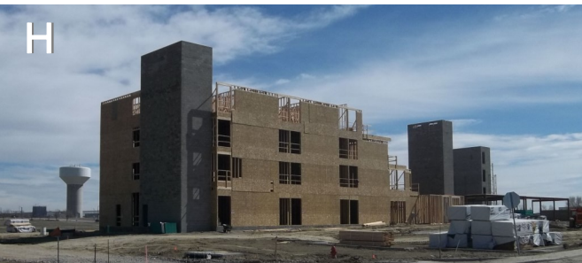
H Eagle Crossing 3rd Filing Subdivision - Spring Hill Suites Hotel - under construction
