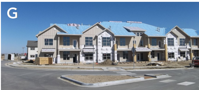
G Highland Meadows Golf Course 12th Filing - 12 unit condo building under construction
