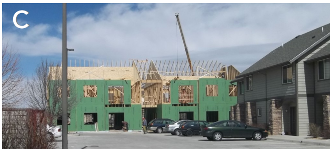
C Grasslands Subdivision 2nd Filing, Lot 1 – 56 unit apartment complex under construction
