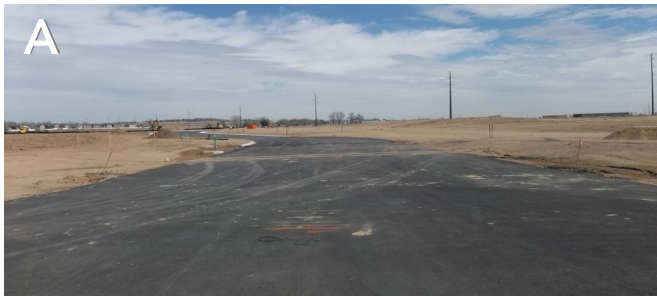
A East Pointe Subdivision –8 lot commercial subdivision under construction—roads and utilities complete
