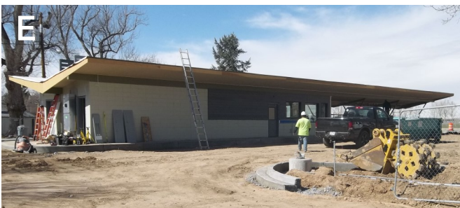
E Homesteaders Landing Subdivision - Dutch Bros Coffee - renovation of existing property
