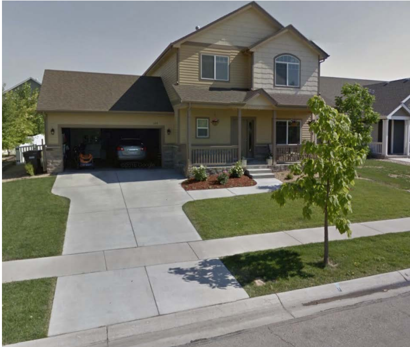
Limited Access: recessed garage. New Windsor
