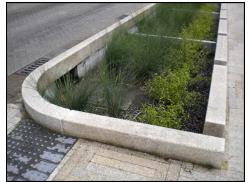
Fig. 3-26-BB: LID stormwater management feature
