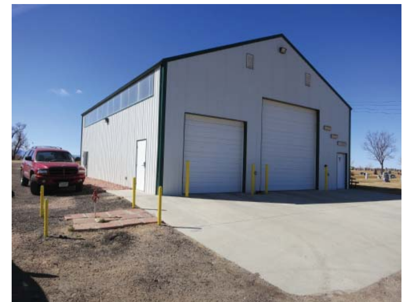
Figure 47: Existing Maintenance Building.
