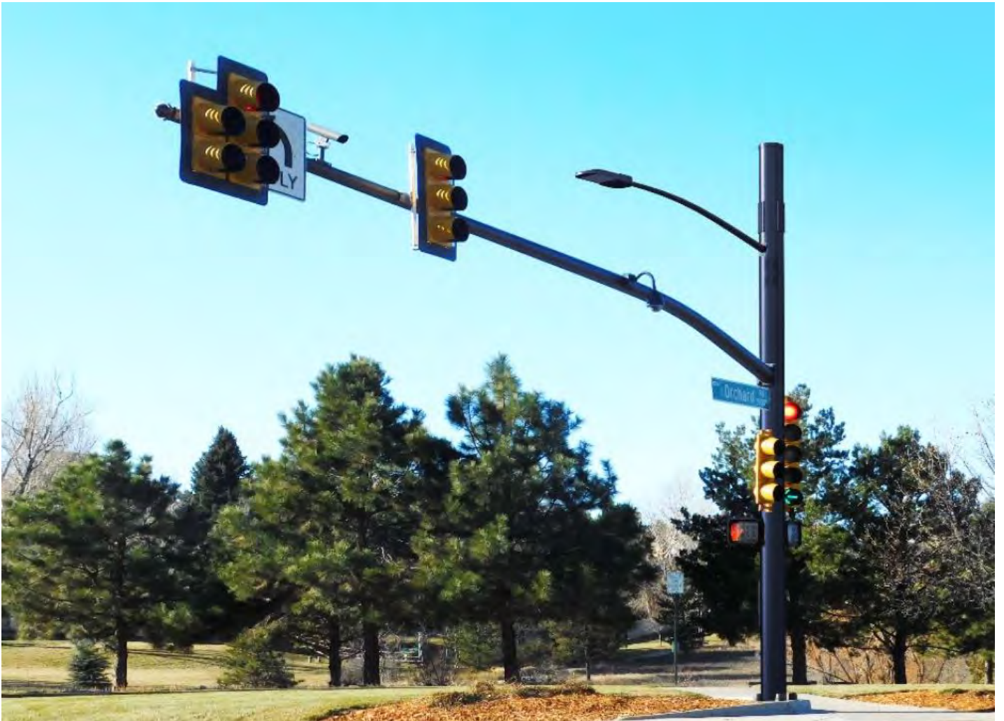
Figure 11: Example traffic signal mounted small cell
