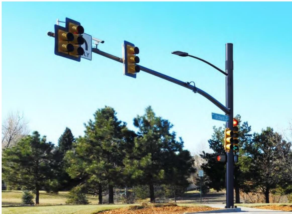
Figure 11: Example traffic signal mounted small cell
