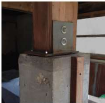
CONCRETE BASE WITH METAL FASTENERS
