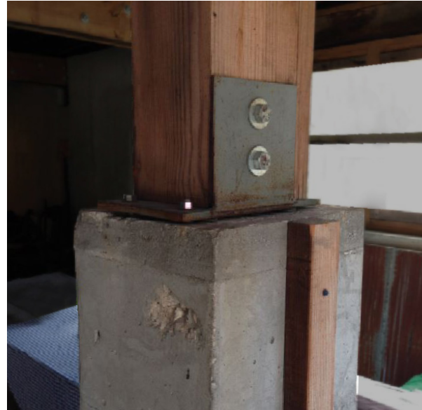
CONCRETE BASE WITH METAL FASTENERS
