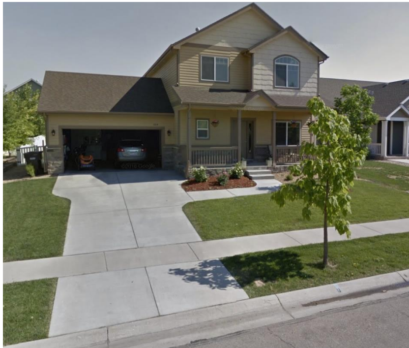
Limited Access: recessed garage. New Windsor
