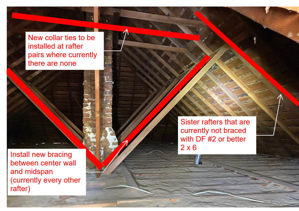
6 ROOF STRENGTHENING DETAIL
