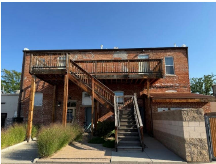
The south-facing side of the building. Flat red brick wall with wooden staircase accessing to the second floor. The ground level has single doors for access. Two windows cutouts have been boarded up and sealed. The second floor has two single doors. Two 1 over 1 window and two window cutouts that have been sealed and bricked.
