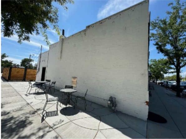
East side of the building with red pressed brick painted white. Descending style roof with a chimney exposed on the south of the wall. Metal plate situated on the lower center.
