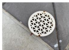
Figure 28 Corrosion around skimmer
