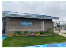
Figure 33 Front of entry building
