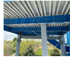
Figure 15 Underside of waterslide tower
