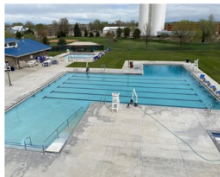
Figure 1 Outdoor Swimming Pool
