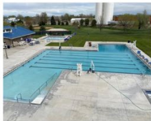
Figure 1 Outdoor Swimming Pool
