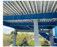
Figure 15 Underside of waterslide tower
