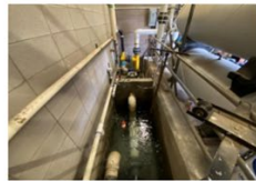
Figure 22 Pool balance tank
