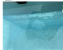
Figure 6 Area of plaster repair, patches
