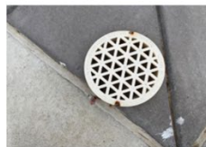
Figure 28 Corrosion around skimmer
