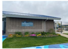
Figure 33 Front of entry building
