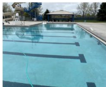
Figure 5 Pool surface staining, etching
