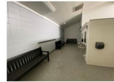
Figure 36 Women's locker room
