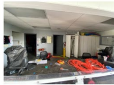
Figure 35 Front entry area
