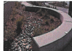
Cast in place concrete boatwall
