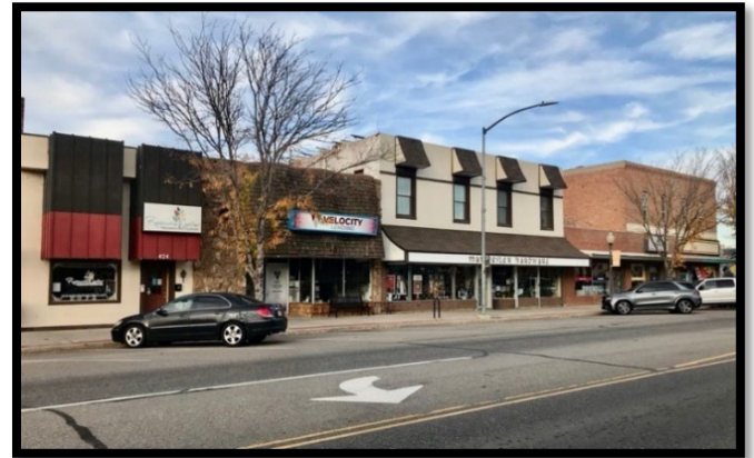
Main Street Commercial Buildings, 400 Block, South Side
