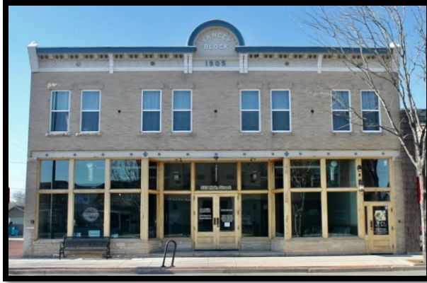
515 Main St., Yancey Block Built 1905
