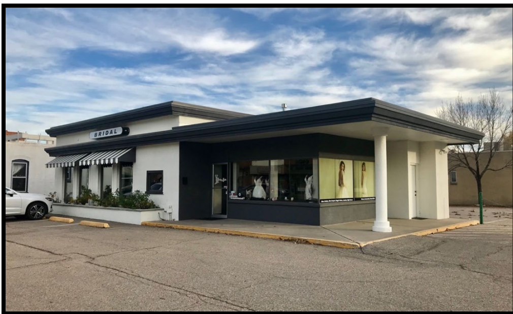
Frontier-Husky Gasoline Station, 529 Main St.
