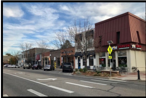
Main Street Commercial Buildings, 400 Block, South Side
