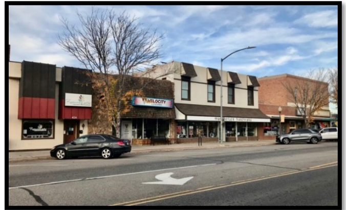
Main Street Commercial Buildings, 400 Block, South Side
